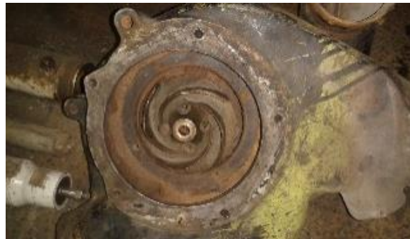
Figure 2: View from the pump's upper cover
