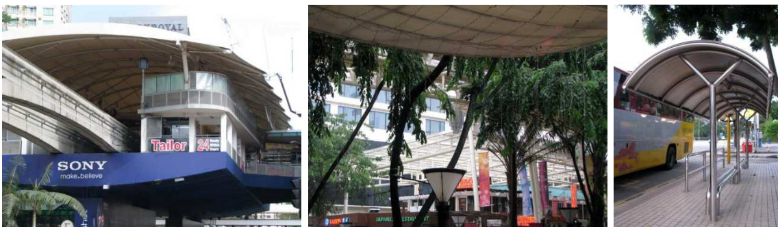
Fig. 17. Using light color materials with low thermal mass in station as a sunshade
