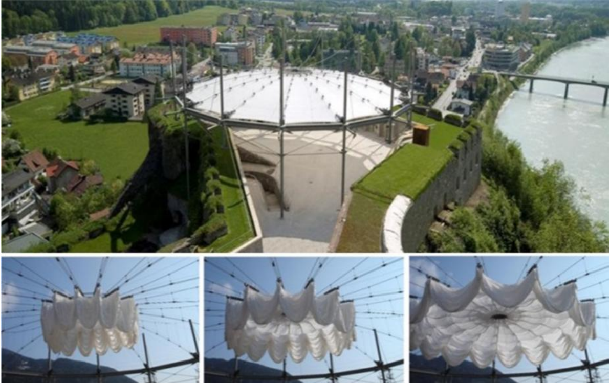
Fig. 04 Fortress Kufstein retractable roof in Austria.
