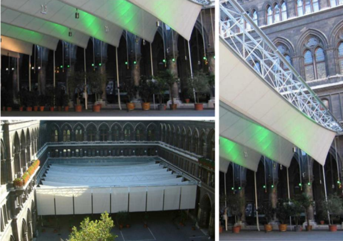
Fig. 03 Town Hale retractable roof in Vienna.
