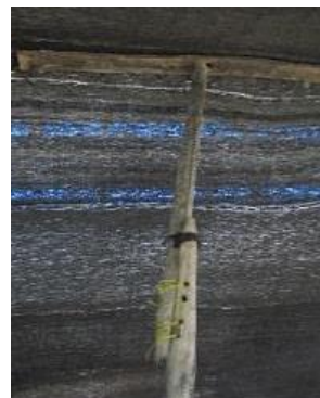
Fig 16. The central column of Arkovazi tent and ridge beam seated on the top of it. The construction covered with the roof fabric (Source: Author)
