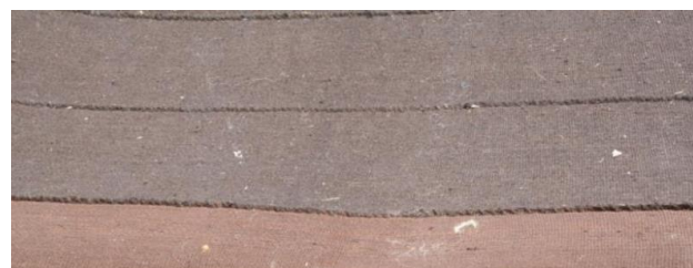
Fig 3. Narrow strips of Black Tent roof cover are sewn together and while on the roof, the seams are parallel to the ridge of the roof; Qashqai Tribe, Fars Province (Source: Author)
