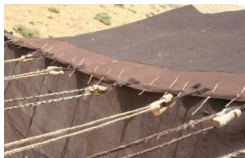
Fig 49. Wall and roof of the tent are connected by wooden pins (Source: Author)
