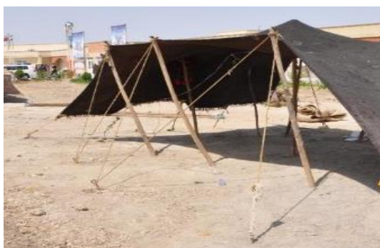
Fig 29. Bahlooli Tribe. Spiral rope between pins and columns (Source: Author)
