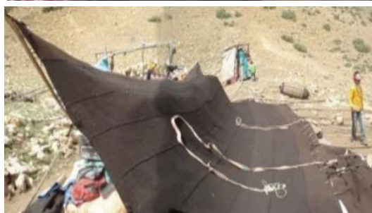
Fig 39. Connection of tent corner to the wooden hook (Source: Author)
