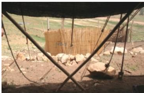
Fig 47. The posts are arranged along the walls of the tent in a criss-crossed way (bracings) (Source: Author)
