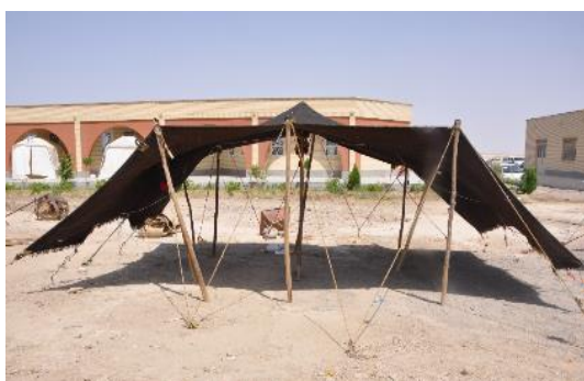
Fig 30. Bahlooli Tribe. View of a Black Tent cover and position of its columns (Source: Author)
