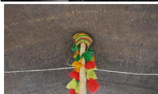
Fig 28. Inside the tent and the placement of columns. Small pillow or pieces of fabric are located between roof cover and column (Source: Author)
