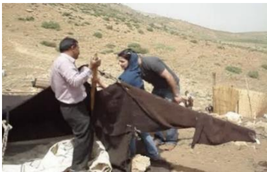
Fig 41. Qashqai Tribe in Fars Province. Pitching the roof by lifting end columns (Source: Author)
