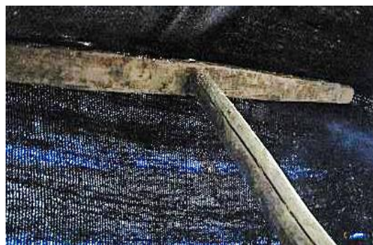
Fig 23. Yarom Tatli Tribe. The central column of the tent and its pass from the carrier beam, to slope the tent (Source: Author)
