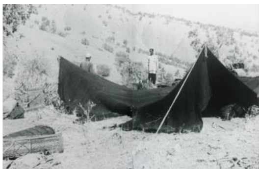
Fig 42. The end corner columns are lifted. [9]
