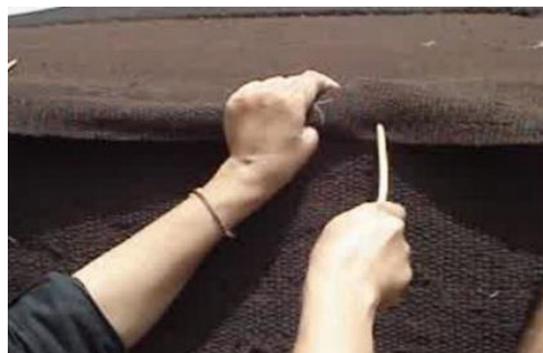
Fig 50. Piercing the cover with thin pins in roughly 20 cm distances to brace the edge (Source: Author)
