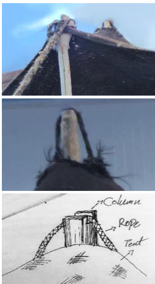
Fig 25. Garapapakh Tribe. The columns are forked at the top and keep a stretching rope attached. The incision on the top of the column keeps the loop sewn on the top of the fabric (Source: Author)
