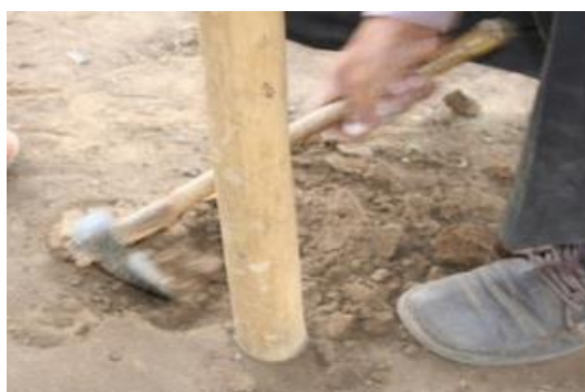
Fig 46. Digging the end column into the ground (Source: Author)
