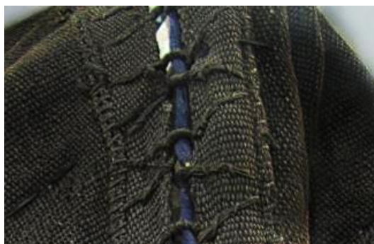
Fig 22. Yarom Tatli Tribe. Method of connecting two parts of the roof (Source: Author)
