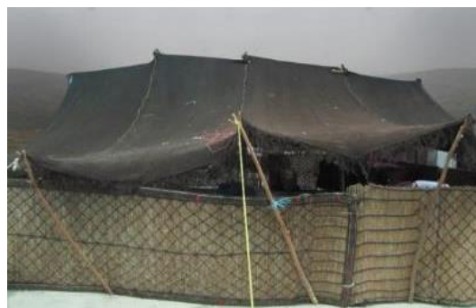
Fig 32. Soleimani Tribe. Four parts of the tent's roof cover are joined by the metal pins (Source: Author)
