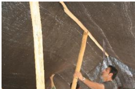
Fig 44. Lifting the middle column with the ridge beam (Source: Author)
