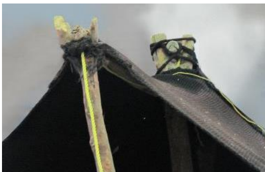
Fig 35. Soleimani Tribe. columns with forked tip form and location of the ridge beam on its (Source: Author)
