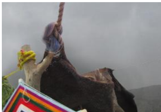
Fig 18. Forked ending of a post with supporting ropes stretching the roof sheet (Source: Author)
