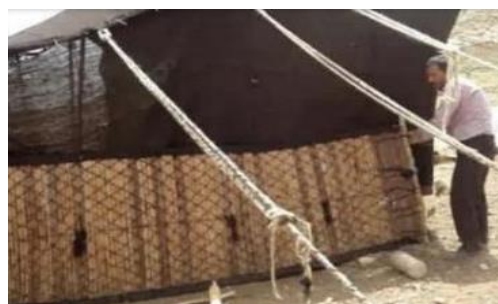
Fig 51. Ramming/pounding into the ground thin branches and unwinding Chigh to support the wall (Source: Author)
