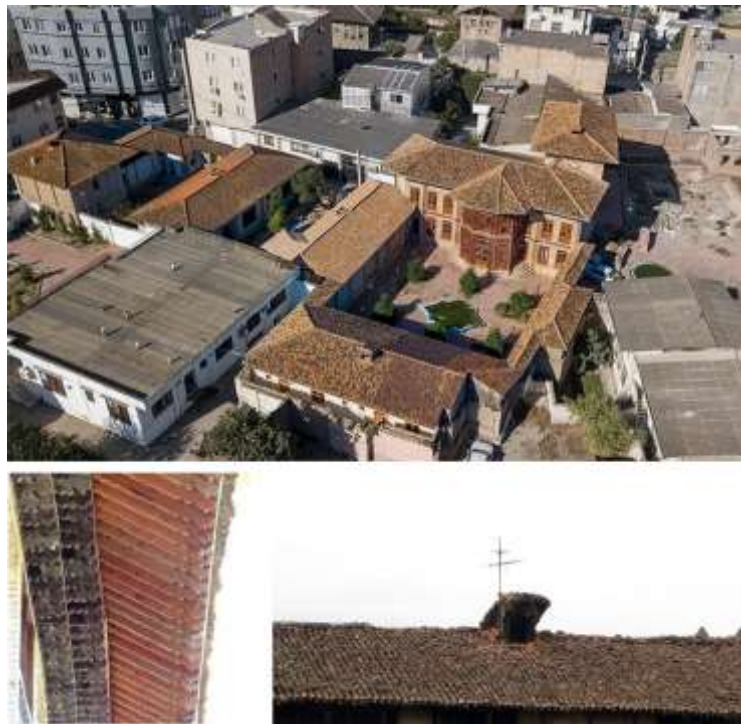
Fig 4. top: cantilevered hip roofs in Sari (Fazeli house); below-left: an example of a three-step "Shir-sar" in Hezarjaribi house; below-right: a typical example of a "Koterkum"
