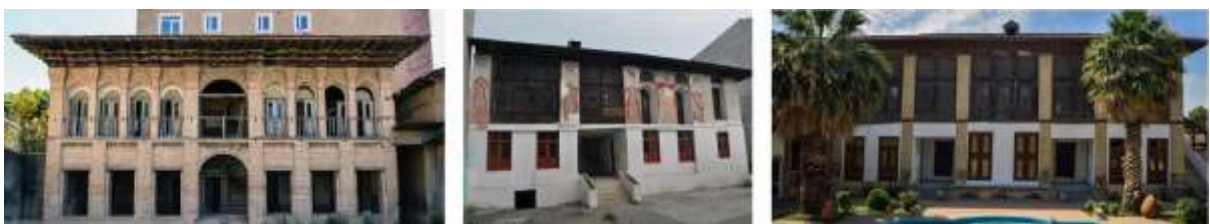
Fig 11. Types of entrance location in the façade. Left: an entrance on the main axis of symmetry which was usually inspired by the European architecture of the time (Sadeghian house), center: an entrance out of the axis of symmetry (Ghoreishi house), right: two entrances located symmetrically (Kolbadi house).
