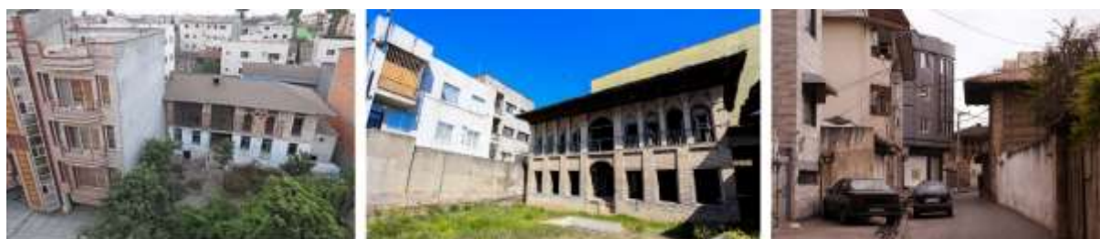
Fig 2. Valuable historical houses surrounded by inharmonious new buildings; left: Ghoreishi house (Amol); middle: Sadeghian house (Sari), right: Ramedani and Mirgati houses (Sari).
