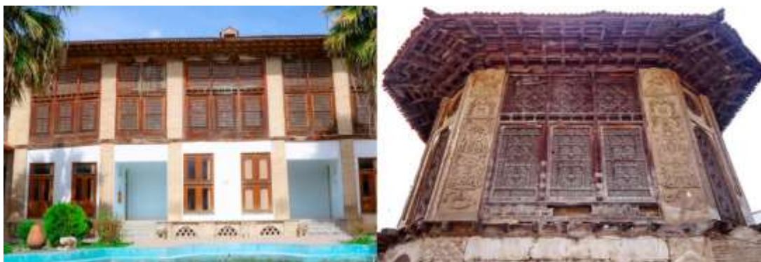
Fig 7. Examples of 'Orosy', the most exquisite openings were used for the most important rooms of the house. Left: Kolbadi house, right: Shafahi house
