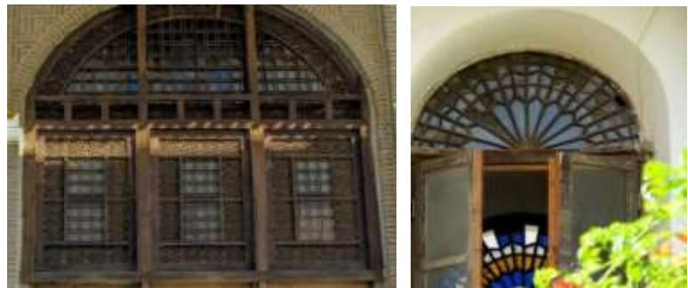
Fig 9. Examples of wooden decoration of window sashes, left: Ramedani house, right: Aghajan-nasab house
