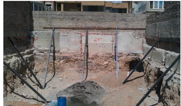
Fig. 7 Photo of excavation
