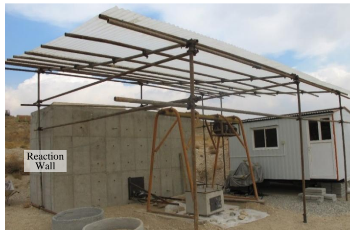
a. Field Laboratory Facility
