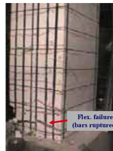
(b) Beam CFB6
