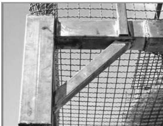
Fig.10 Using corbels for strengthening the connections
