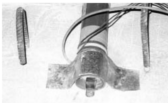
Fig. 7. Fixing the head of the pipe on the pedestal
