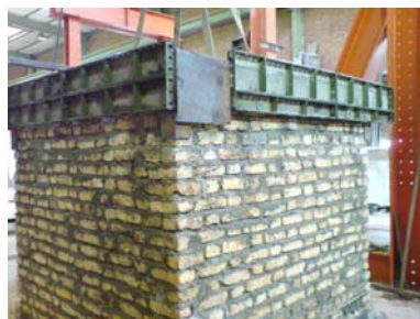
c) Reinforcing and concreting of slab and upper tie
