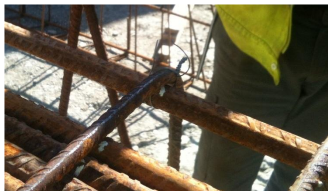
Fig. 5 Close-up of mechanical tying
