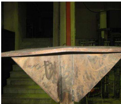
Fig. 25 Sagged plate near the connecting bolt
