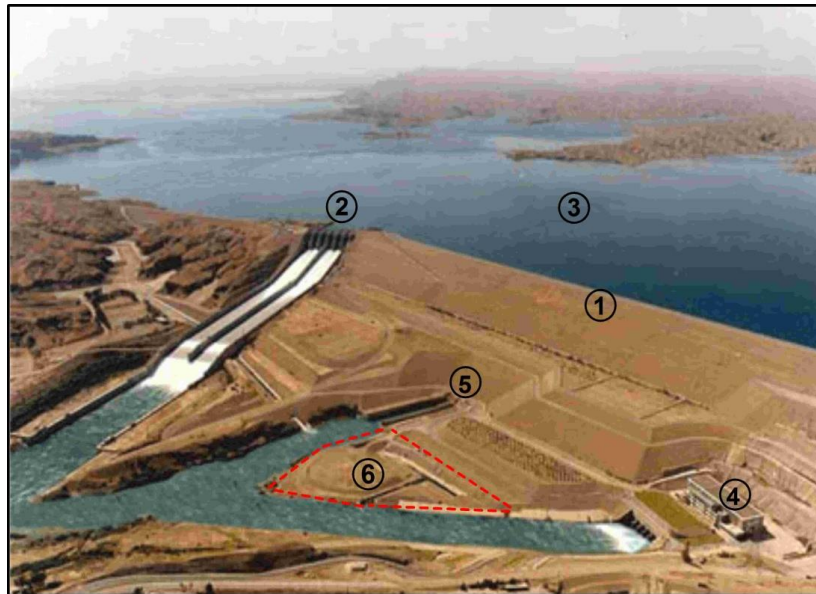
Fig. 1 General plan of the Karkheh dam project. The numbers represent: 1, dam crest; 2, spillway; 3, reservoir; 4, powerhouse; 5, diversion culverts; and 6, the location of the new relief wells at dam toe (the red-dashed polygon)
