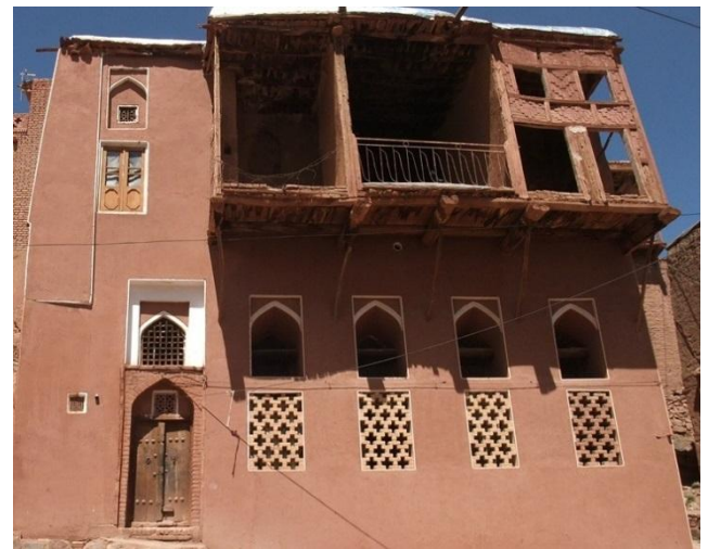
Fig. 3 A view of a three story historical building in Abyaneh
