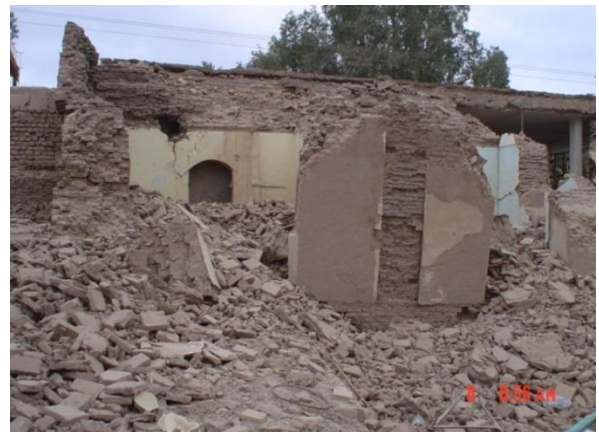
Fig. 1 A view of one sample destroyed adobe house after Bam earthquake
