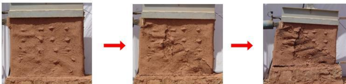
Fig. 15 Damage mechanism of RMW1 wall
