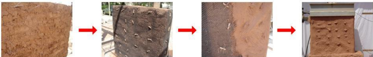
Fig. 14 Installation process of polypropylene lace on adobe walls
