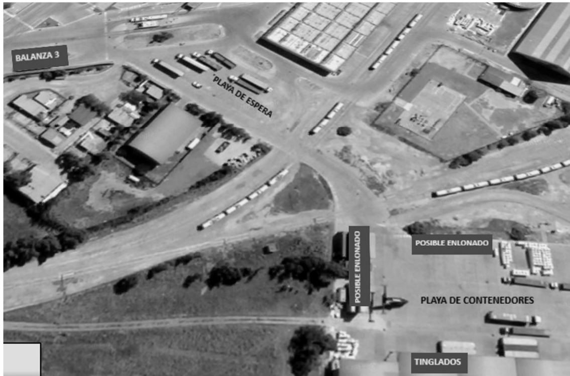
Fig. 4. Possible places for truck covering place.
